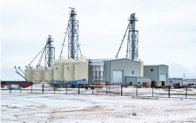
Seed cleaning plant under construction 2023
